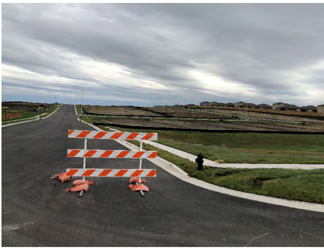
Entry road to Phase I
