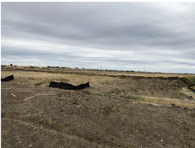
Land under construction in Phase II
