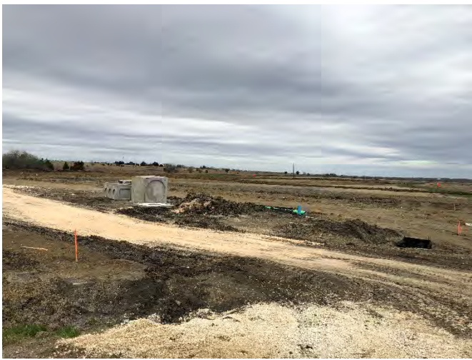
Interior view of construction in Phase II
