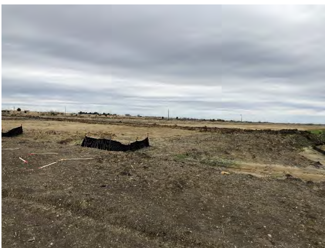
Land under construction in Phase II
