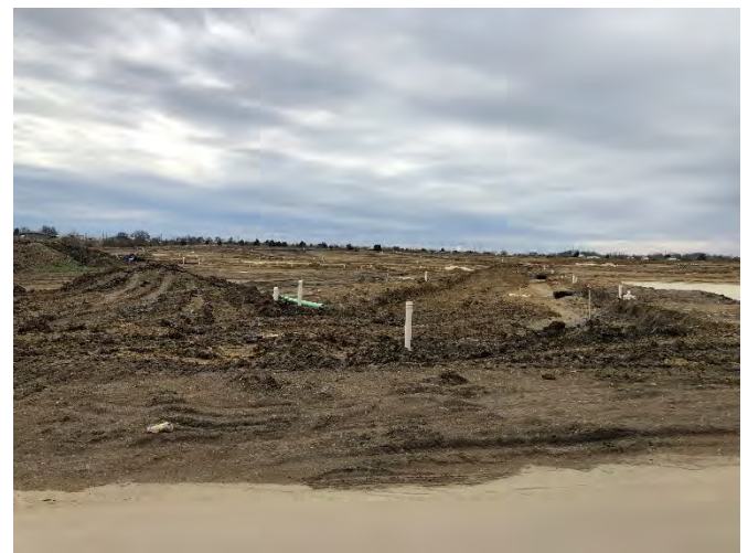
Land under construction in Phase II
